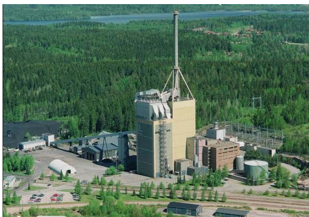
Figure 2.4: The Kymijärvi power plant with biomass gasifier, at Lahti
