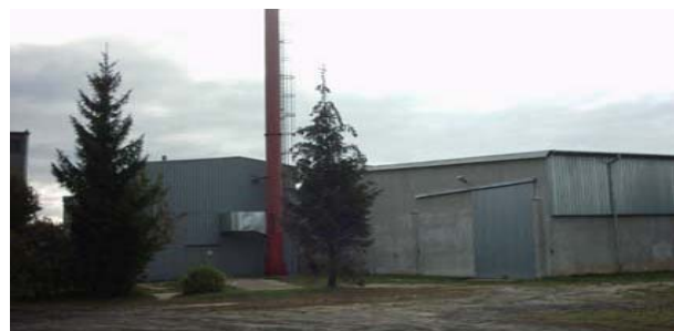
Figure 2.3: The straw-fired heat plant in Przechlewo
