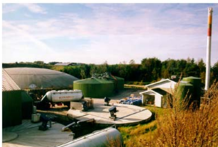
Figure 2.8: The Vaarst-Fjellerad biogas plant
